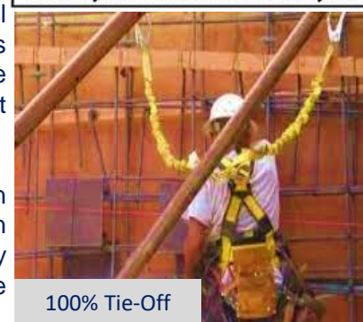
Full-Body Harness and Fall-Arrest System
